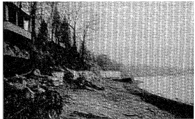
Erosion of bluffs overlooking the Great Lakes has caused an immediate hazard to many lakefront homes. Some were certified as being in danger of imminent collapse and were eligible for federal assistance under Upton-Jones to be relocated.
