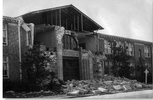
Seismic shaking primarily affects unreinforced masonry buildings, as seen here with this Long Beach middle school damaged by the 1933 Long Beach earthquake. Image from Los Angeles Times.
