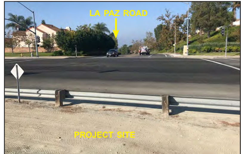
D. Looking at future site access at La Paz Road and Olympiad Road
